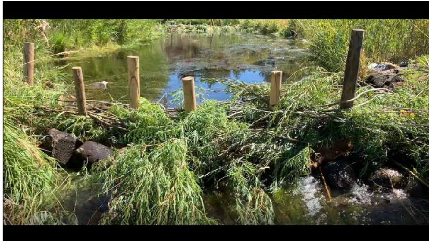
Beaver Dam Analogs (BDAs) are built by pounding posts into the substrate and weaving in willows and shrubs, placing rocks and mud to create a semi-permeable structure. Photo: Swaner Preserve
