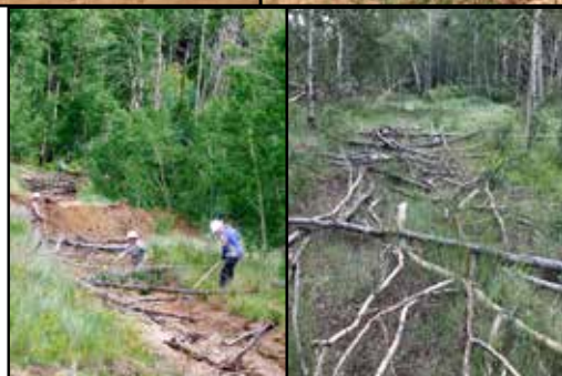
Large berms and cable fences at the closure, placing logs and brush to reduce erosion, vegetation in 2018.
