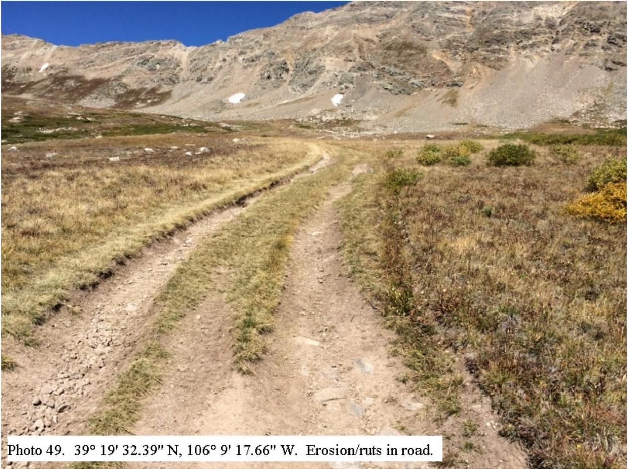
Photo 49. 39° 19' 32.39" N, 106° 9' 17.66" W. Erosion/ruts in road.
